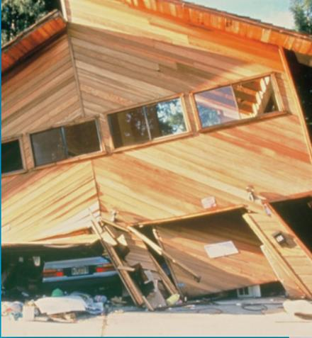
The walls around the garage door of this home were not strong enough to withstand the shaking of the 1989 Loma Prieta Earthquake.
