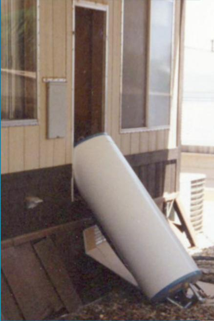
*During an earthquake, an unbraced water heater can topple, which can start a fire or lead to major water damage.*
