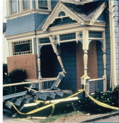
This older home collapsed after earthquake shaking damaged its crawl space (cripple) walls.
