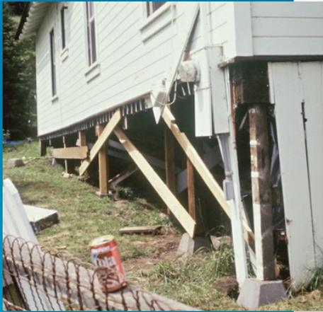
This home's pier-and-post foundation was damaged during an earthquake. The diagonal bracing was added after the earthquake to temporarily stabilize the home during repairs.
